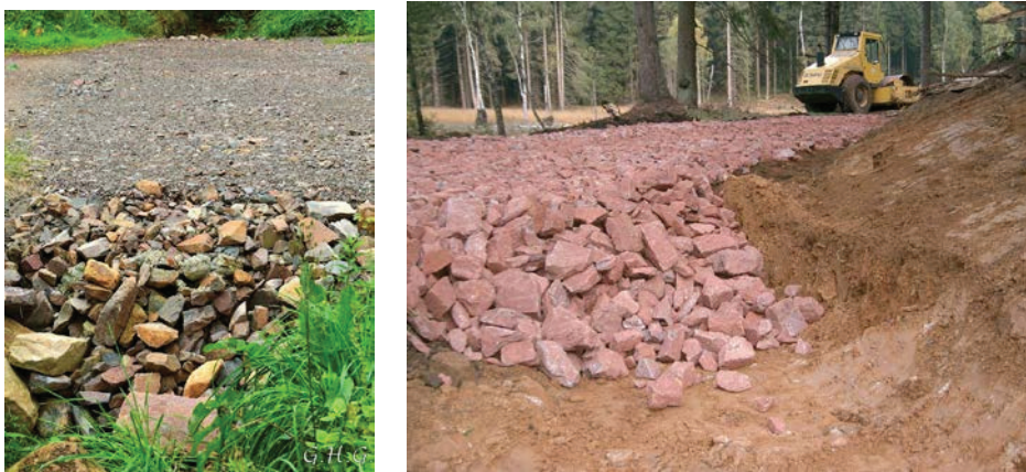
Figure 54 - Covering of forest road with rocks, gravel
